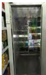
A curtain installed in a walk-in refrigerator
